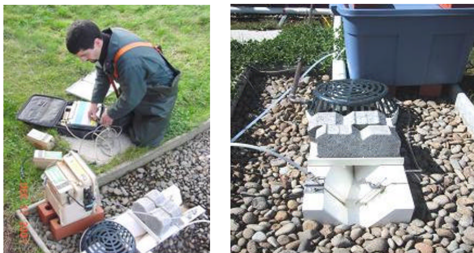
Figure 8 . Two photographs of one of the monitoring stations. One shows the data logger and bubbler with the flume and the second is a close-up of the flume.
