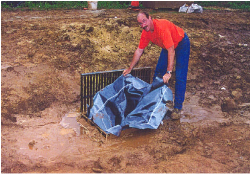
Figure 1 – Example of Type 1 Geotextile Catch Basin Insert -- Siltsack ® by ACF Environmental
