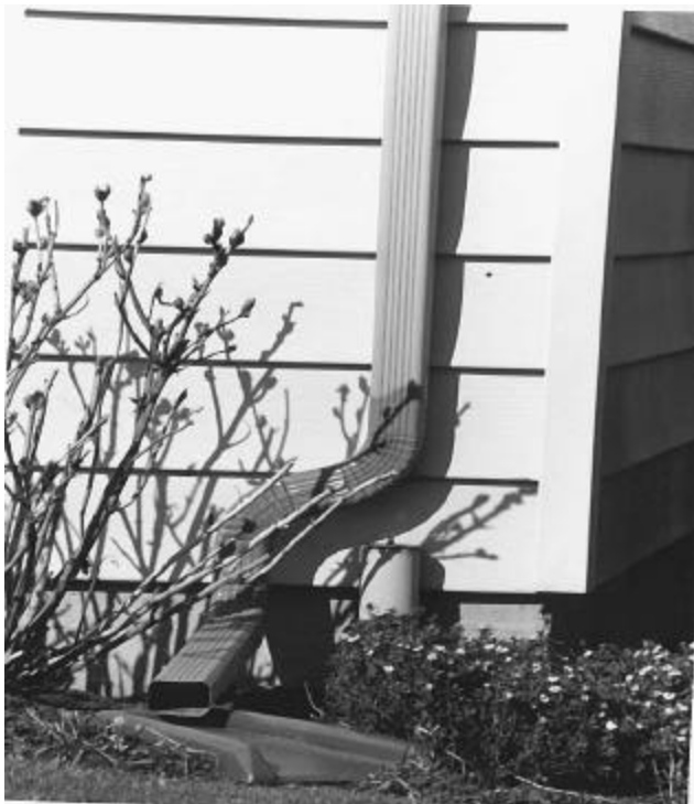
(Figure No. 3) Typical Residential Downspout Disconnection
