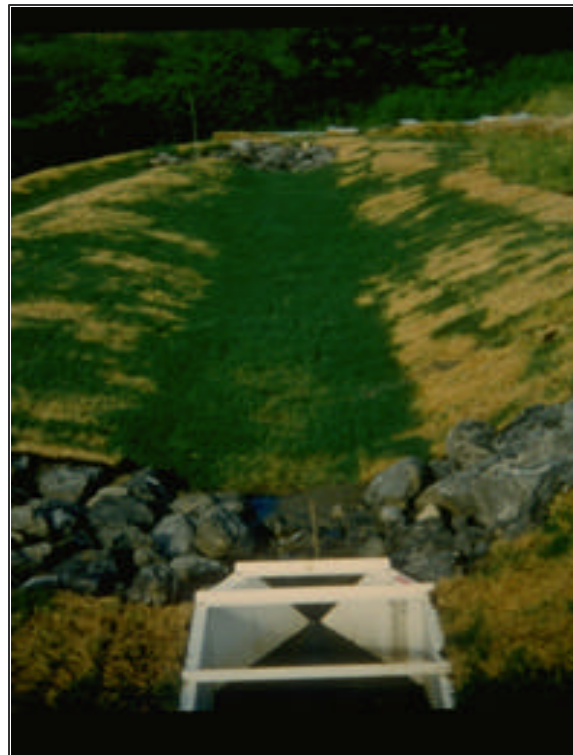
Figure 5- Swale (courtesy of Hydro Compliance Management, Inc.)
