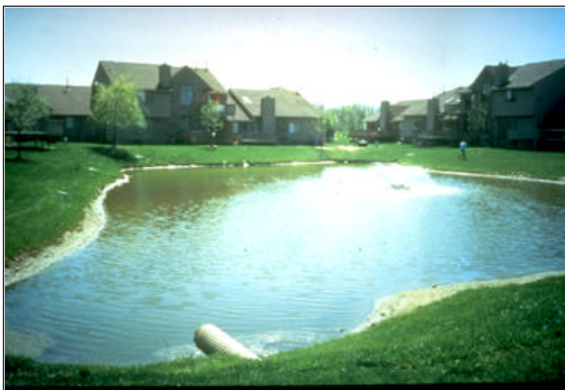
Figure 3- Wet Pond (courtesy of Hydro Compliance Management, Inc.)
