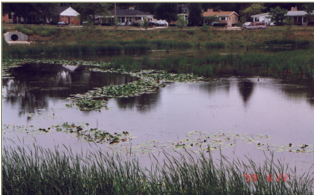
Figure 4 -Example of constructed wetland -- Tollgate Storm water Treatment Facility Lansing, Michigan (courtesy of Patrick Lindemann, Ingham County Drain Commissioner, and designer of the project)
