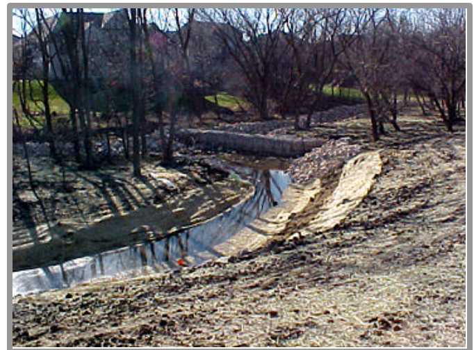
Figure 8. A rock lined channel provided rapid infiltration of runoff, substantial heat dissipation, and near complete control of channel erosion. Rock-filled gabion dams located near channel restrictions provided easily accessible maintenance sites. Sediment and debris that accumulated upstream from the dams could be readily removed in these areas. The rock dams filtered large sediment and debris, slowed the flow of water, and dissipated heat.
