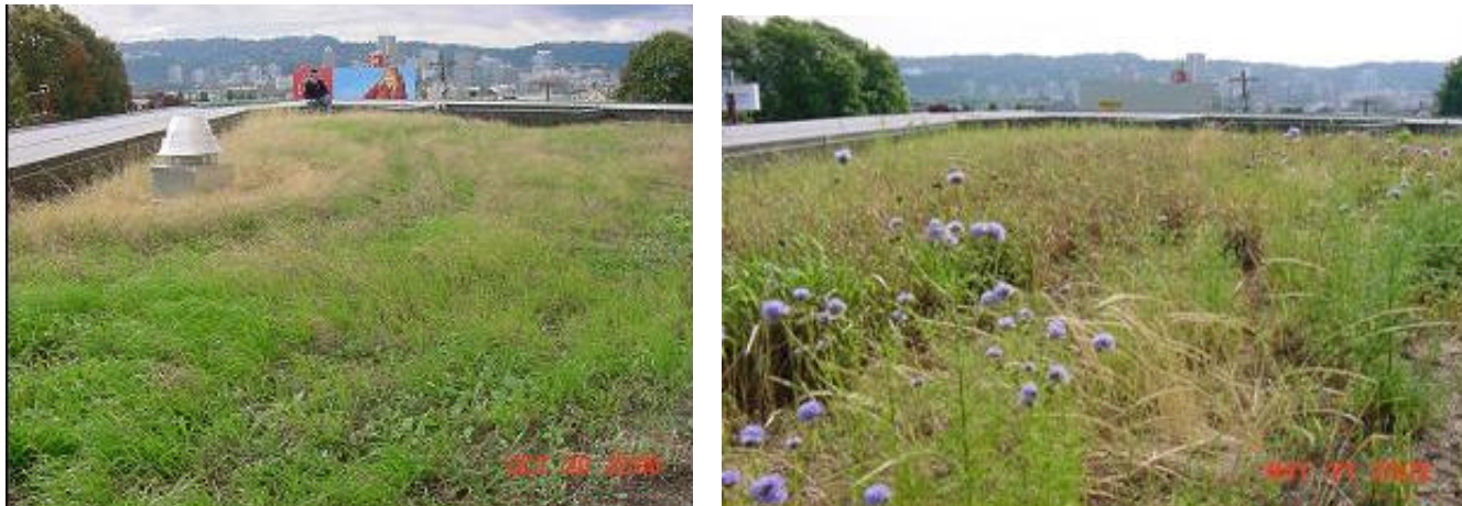
Figure 14. Two photographs of the Buckman Terrace EcoRoof showing uses of grasses and wildflowers.
