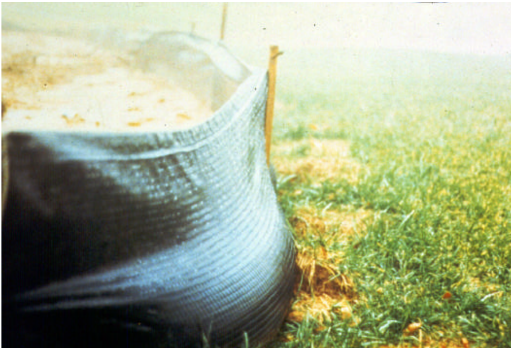
Figure 2 – Example of Silt Fence Containing Sediment -- Geotex ® by SI Geosolutions
