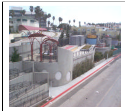
Figure 17. The Santa Monica Urban Runoff Recycling Facility.
