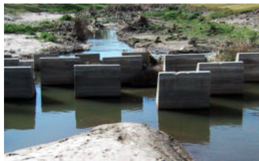
Photo 4 – San Diego Crk looking downstream from grade control structure at energy dissipaters.
