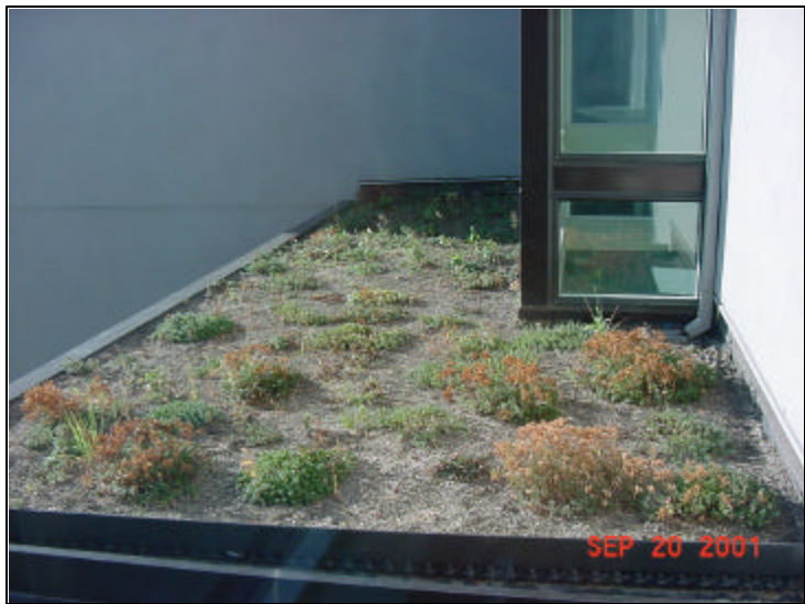
Figure 15. Buckman Terrace EcoRoof at the building entry with protection from north facing wall
