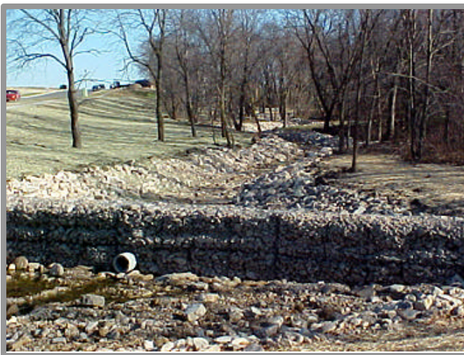
Figure 8. A rock lined channel provided rapid infiltration of runoff, substantial heat dissipation, and near complete control of channel erosion. Rock-filled gabion dams located near channel restrictions provided easily accessible maintenance sites. Sediment and debris that accumulated upstream from the dams could be readily removed in these areas. The rock dams filtered large sediment and debris, slowed the flow of water, and dissipated heat.
