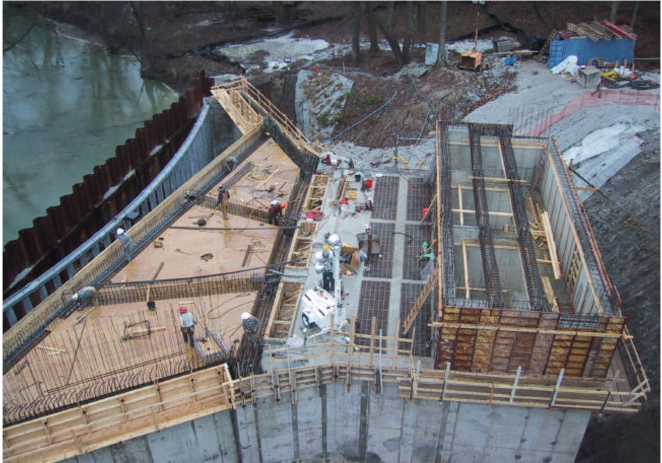
Figure 5. Diversion structure at Thorn Creek during construction
