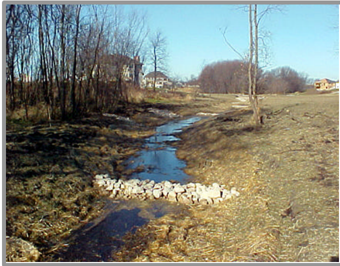
Figure 7. Erosion control matting and a rock check dam combine to reduce stream channel erosion and enhance storm water infiltration in developed headwater areas.
