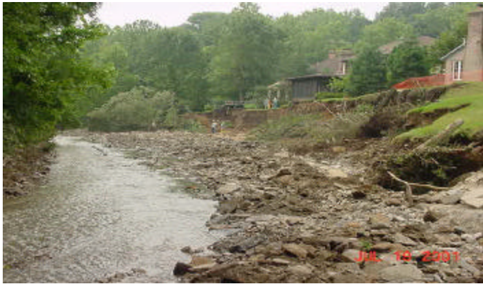
Erosion Damage along Polk Run from storm of July 17— 18, 2001
