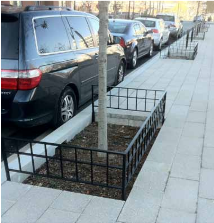
Above: Infiltration tree boxes at Canal Park in Washington DC blend in with the existing streetscape. Security edging and curb cuts blend seamlessly into the street profile.
