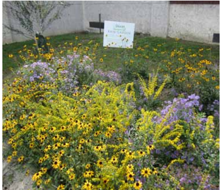
Above: Bioretention basins (i.e., rain gardens) allow rain and snowmelt to seep naturally into the ground while also providing visually appealing landscaping. Below: Water from the roof of a rowhouse in downtown DC is directed towards a backyard rain garden/bioretention basin.
