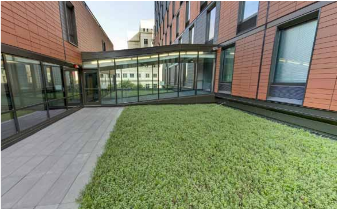
Above: Close-up of an extensive green roof atop of the newly constructed Rutgers dorm. Such systems can significantly extend the amount of time it takes for water to leave a site.
