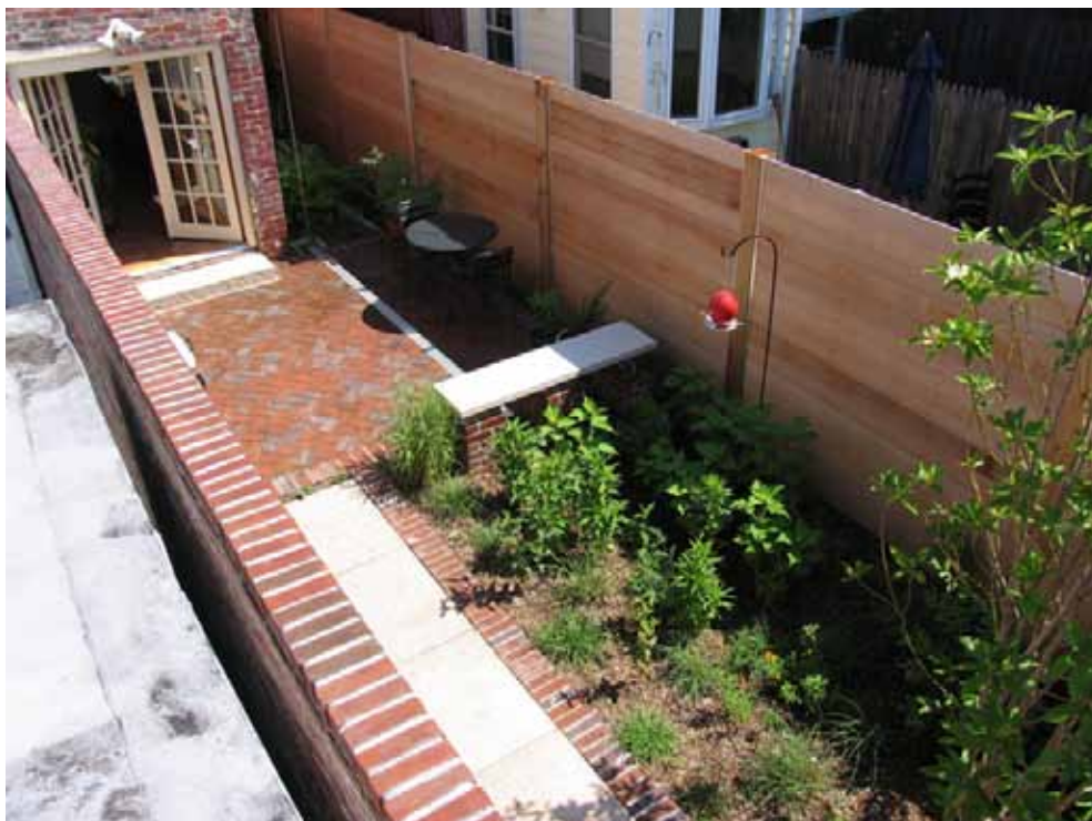
Above: Bioretention basins (i.e., rain gardens) allow rain and snowmelt to seep naturally into the ground while also providing visually appealing landscaping. Below: Water from the roof of a rowhouse in downtown DC is directed towards a backyard rain garden/bioretention basin.
