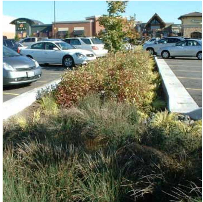
Above: A bioretention swale filters rainwater in a shopping center parking lot. Below: A bioretention swale in an urban park setting.
