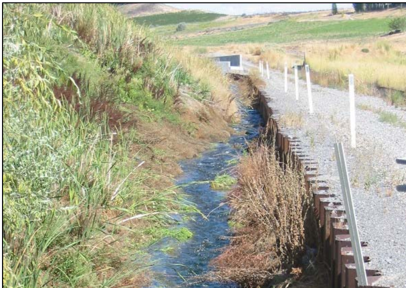
Figure 2. Example of a modified stream. Several indicators are apparent in this reach, but assessor should note the strength of indicators in upstream or downstream segments that are not directly affected by the road. Such field notes will more fully describe the site and may be useful in determining flow duration.
