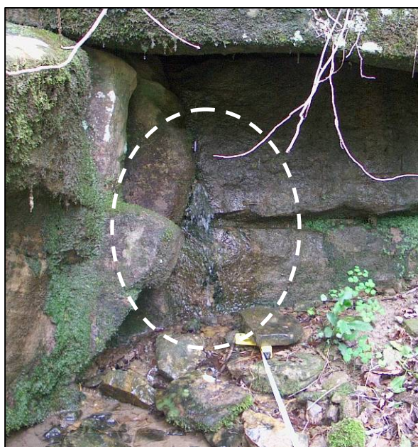
Figure 27. Seep discharging from fractured bedrock on channel margins.
