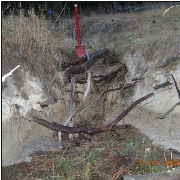
Figure 24. Headcut, viewed from downstream (Blue Mountains, approximate channel width outside of the scour zone is 0.5 m). This is a large feature, given the channel dimensions.
