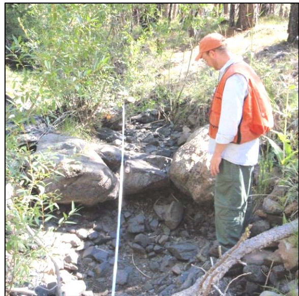
Figure 21. Grade control comprised of very large sediment particles (channel width 2.8 m). This is a medium-sized feature, given the channel dimensions.
