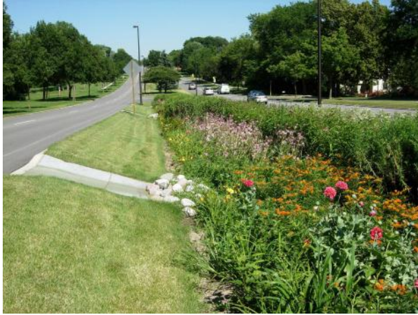
Figure 4-1. Bioretention in Median
