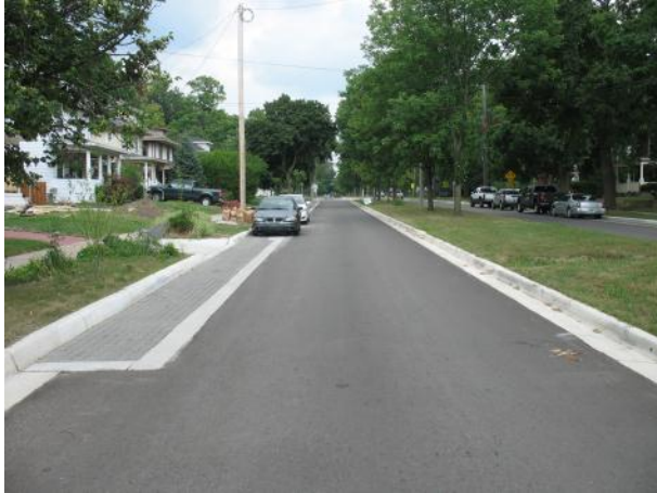
Figure 4-3. Permeable Interlocking Concrete Paver Parking Lane
