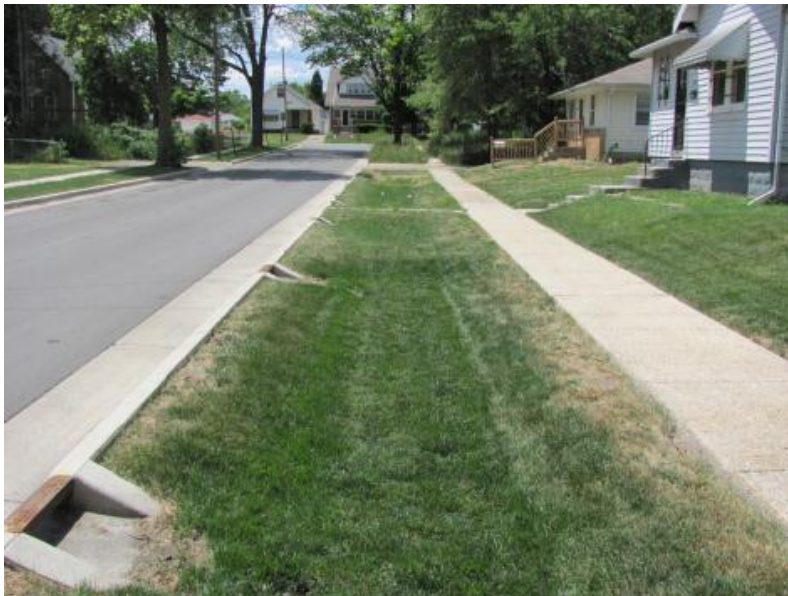
Figure 6-1. Bioretention Planted with Turf Grass
