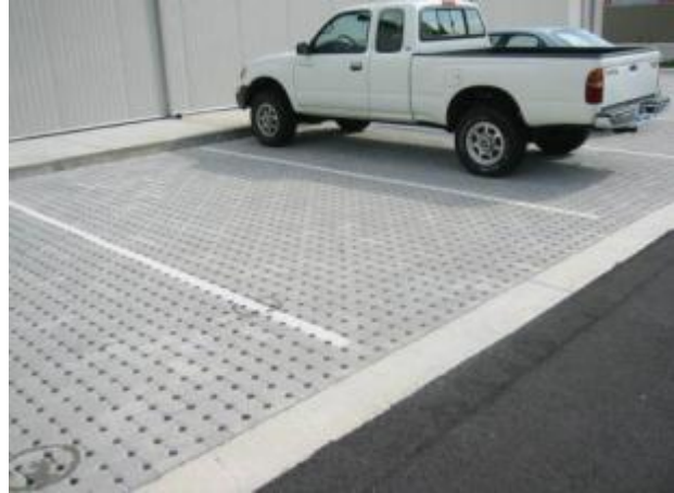
Figure 4-4. Permeable Interlocking Concrete Paver Parking Stalls
