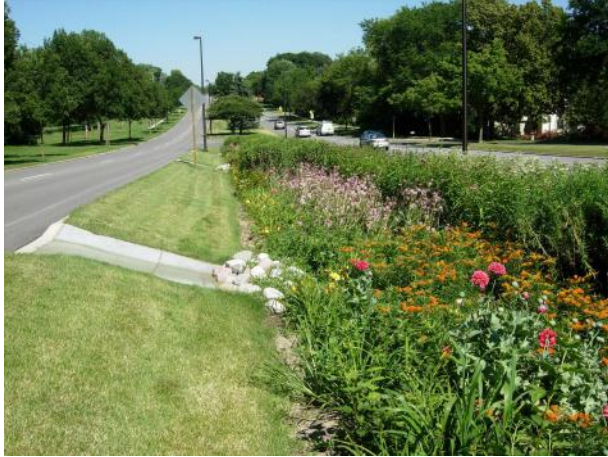
Figure 4-1. Bioretention in Median
