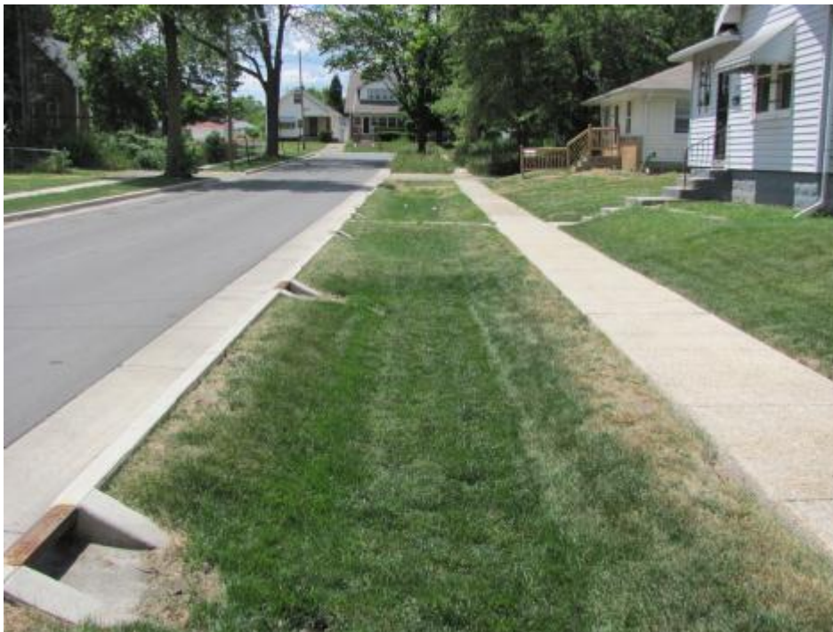
Figure 6-1. Bioretention Planted with Turf Grass
