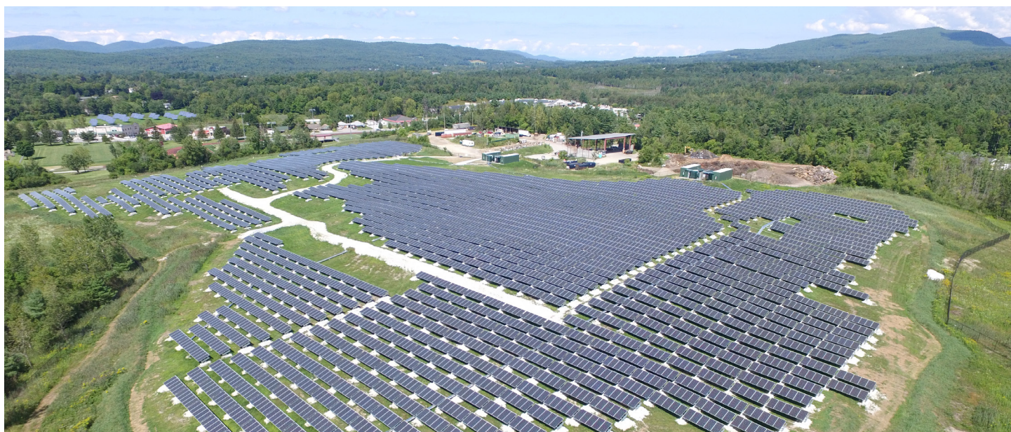
Stafford Hill Solar Farm. Photo courtesy Green Mountain Power.
