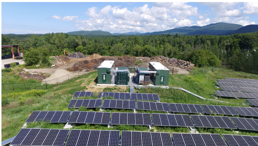
Stafford Hill Solar Farm and battery system. Photo courtesy Green Mountain Power.
