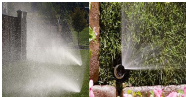
The system on the left is operating under too-high pressure (photo courtesy of Irrigation Association); the right photo shows correct pressure (photo courtesy of Rain Bird).
