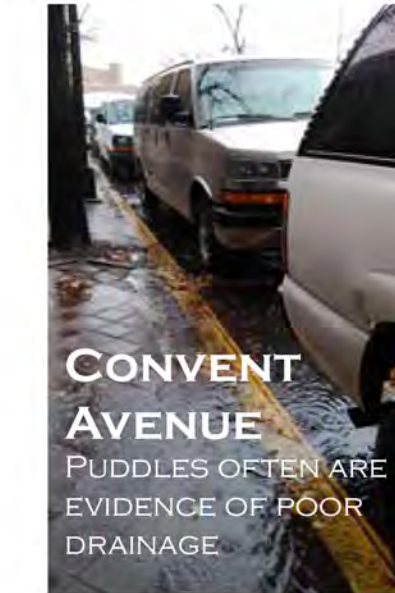
CONVENT AVENUE THESE ROUTINE PUDDLES HAVE ERODED THE SIDEWALK AWAY AFTER YEARS OF FREEZE AND THAW CAUSING TRIPPING HAZARDS.
