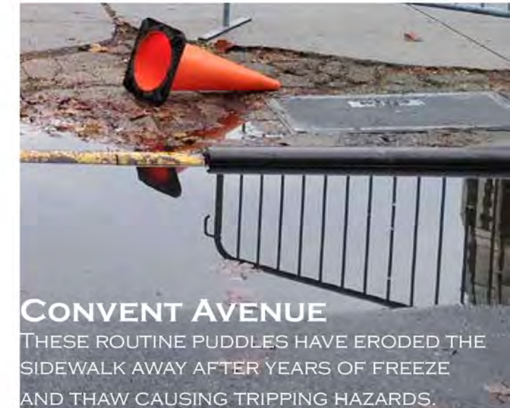
CONVENT AVENUE PUDDLES OFTEN ARE EVIDENCE OF POOR DRAINAGE.
