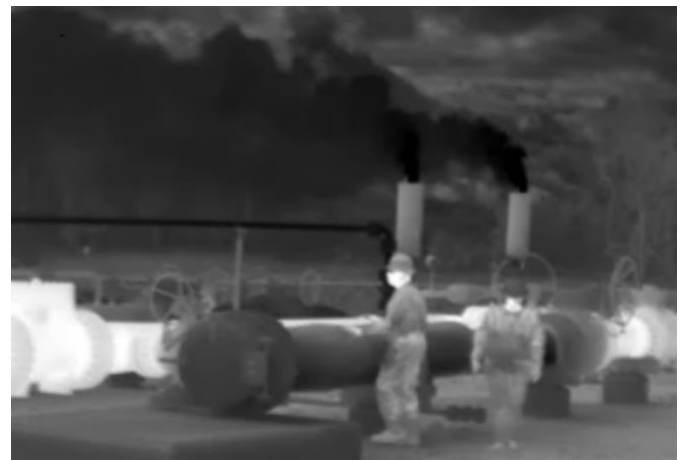
Infrared Image of Compressor Station Pig Receiver Depressurization Event
