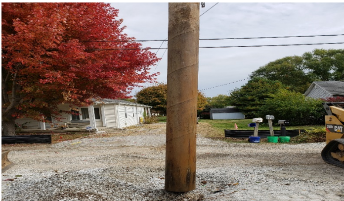
Photo #3: Looking east at dewatering point being removed
