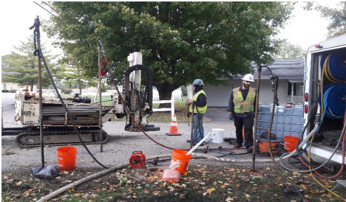
Photo #1: View of Regenesis pilot study injection activities near MW-35
