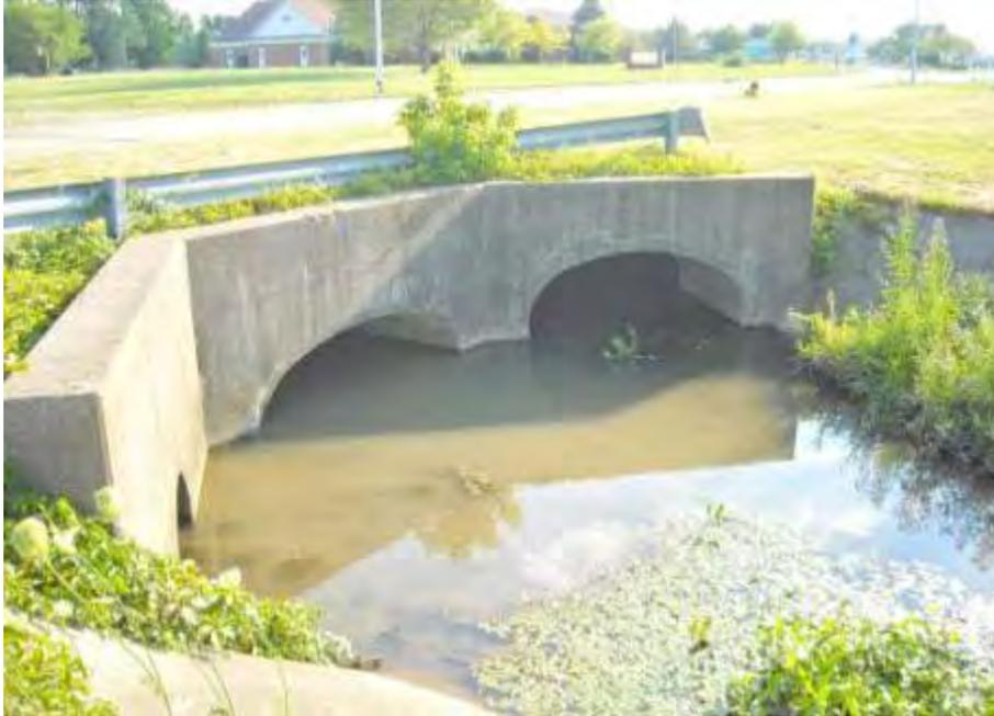
**Figure 3-19** Three large culverts are located immediately upstream of the Amlosch Ditch sampling location (AD-1). The center culvert transmits upstream flow beneath Dustin Road.
