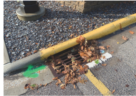
Figure 7: Photo of an Agriculture Mall drain inlet that leads to the combined sewer system
