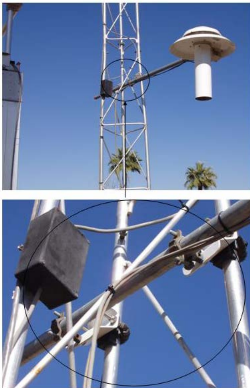
Figure 1.14 Temperature Cable Installation and Expanded/Close-Up Views
