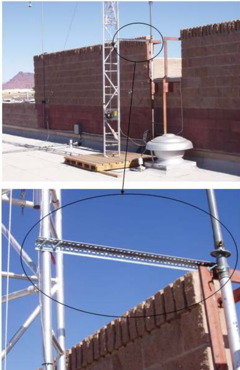
Figure 1.9 (a) Angle Iron Support—Expanded View; (b) Angle Iron Support—Close-Up View
