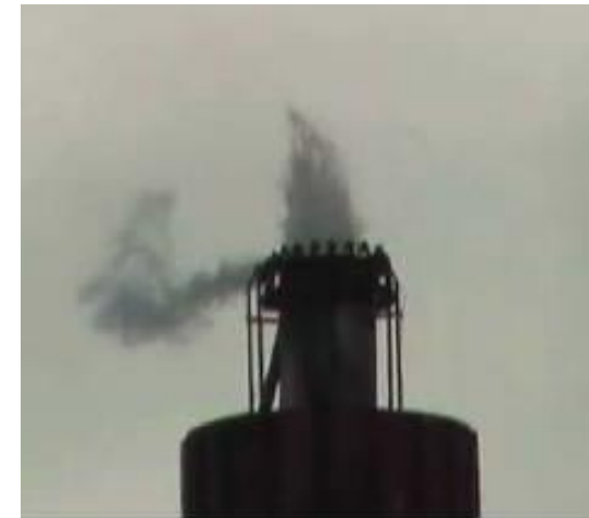
Poorly Operating Flare/Over Steamed – Low Combustion Efficiency
