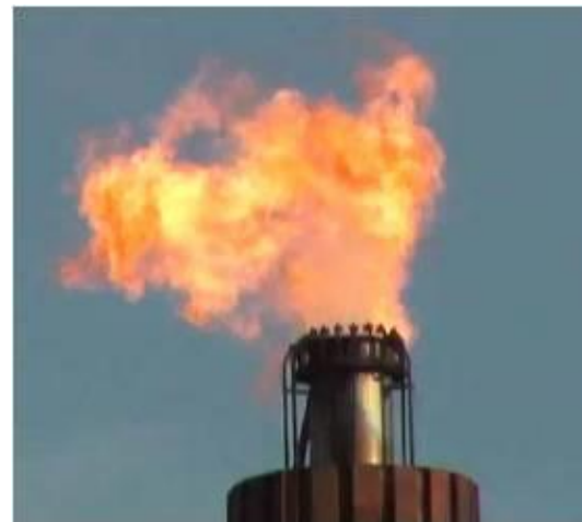
Well Operating Flare – High Combustion Efficiency
