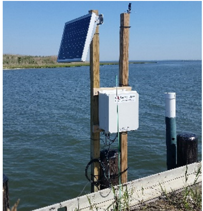
Piling with solar panel at Morrison's Marina, Beach Haven, NJ
