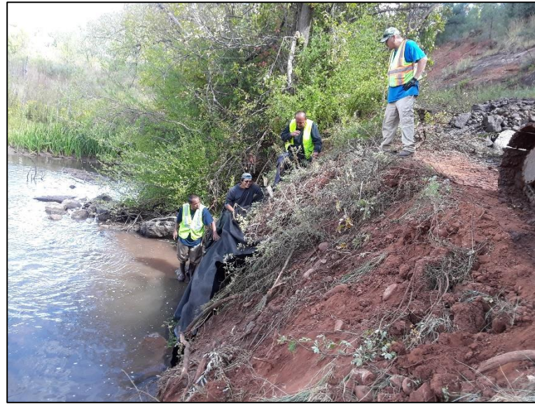
White Mountain Apache. Livestock exclusion fencing and stream stabilization on the North Fork White River.
