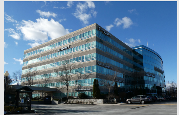
500 Cummings Center achieved ENERGY STAR-certification in 2011. Its tenants include a range of businesses, from medical to financial and more.
