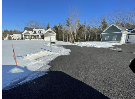
POROUS ASPHALT DRIVEWAY AND POROUS ASPHALT ROADWAY 2/9/2022
