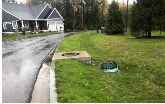
BIOSWALE AND PRETX POST-CONSTRUCTION
