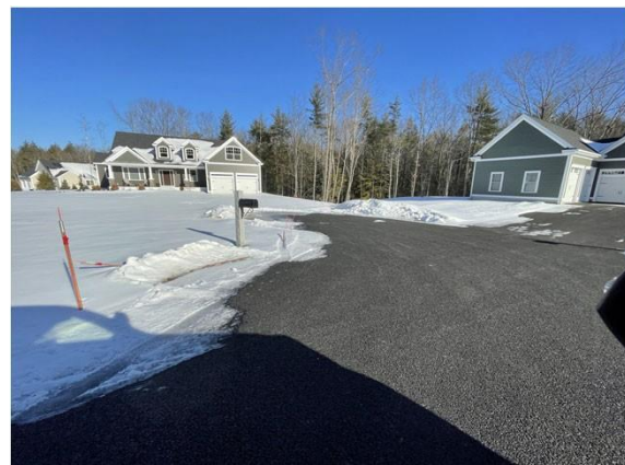
POROUS ASPHALT DRIVEWAY AND POROUS ASPHALT ROADWAY 2/9/2022
