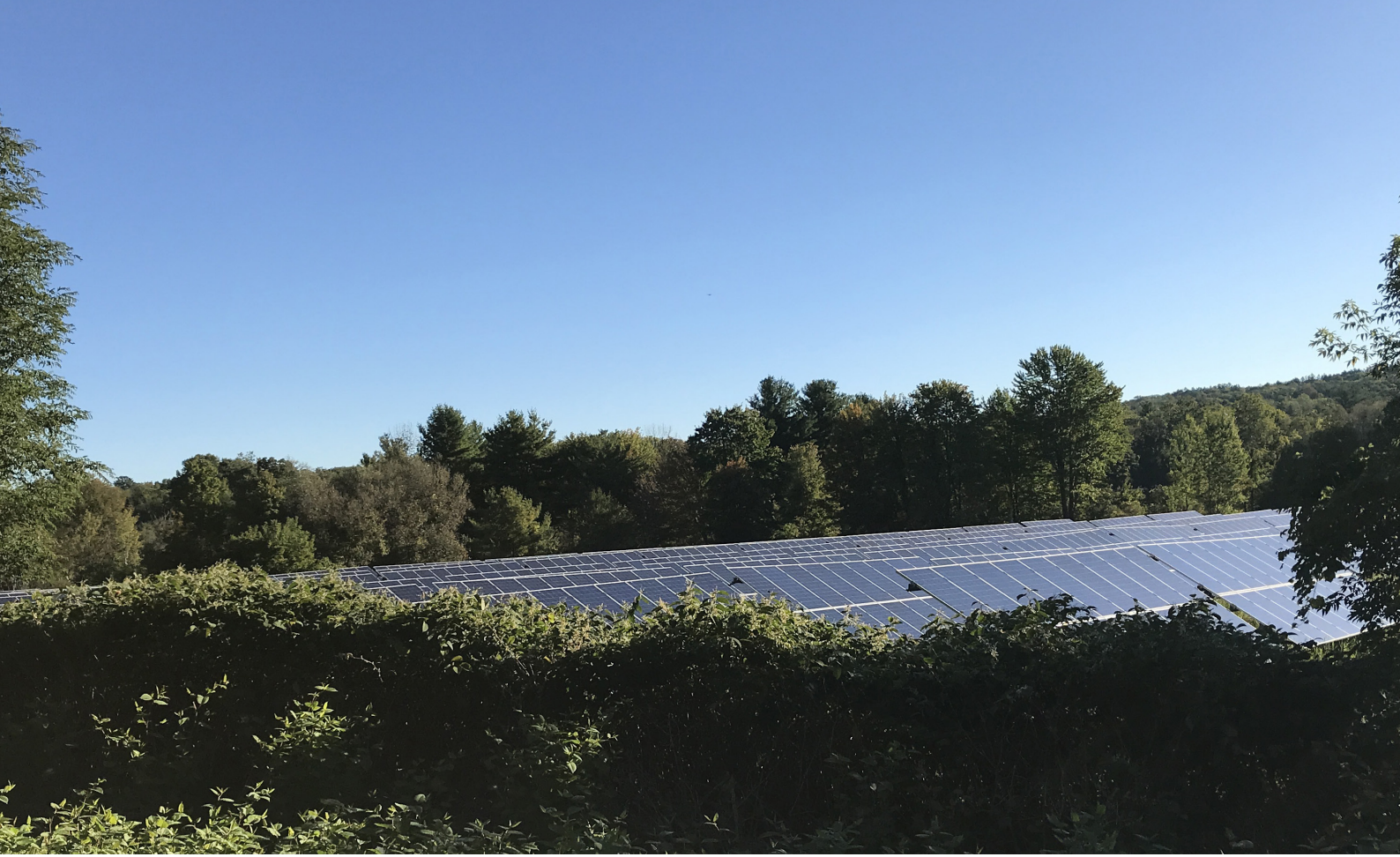
Above: Solar field in the Town of Glenville, Schenectady County, NY
