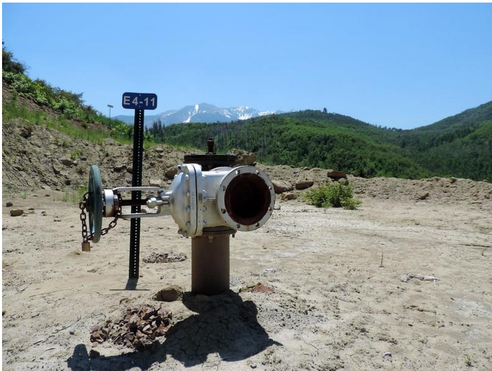
Figure 5: Mine ventilation boreholes are drilled to vent gas into the air from pipes
