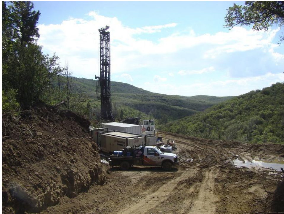
Figure 7: Mine ventilation boreholes require drilling and heavy industrial equipment
