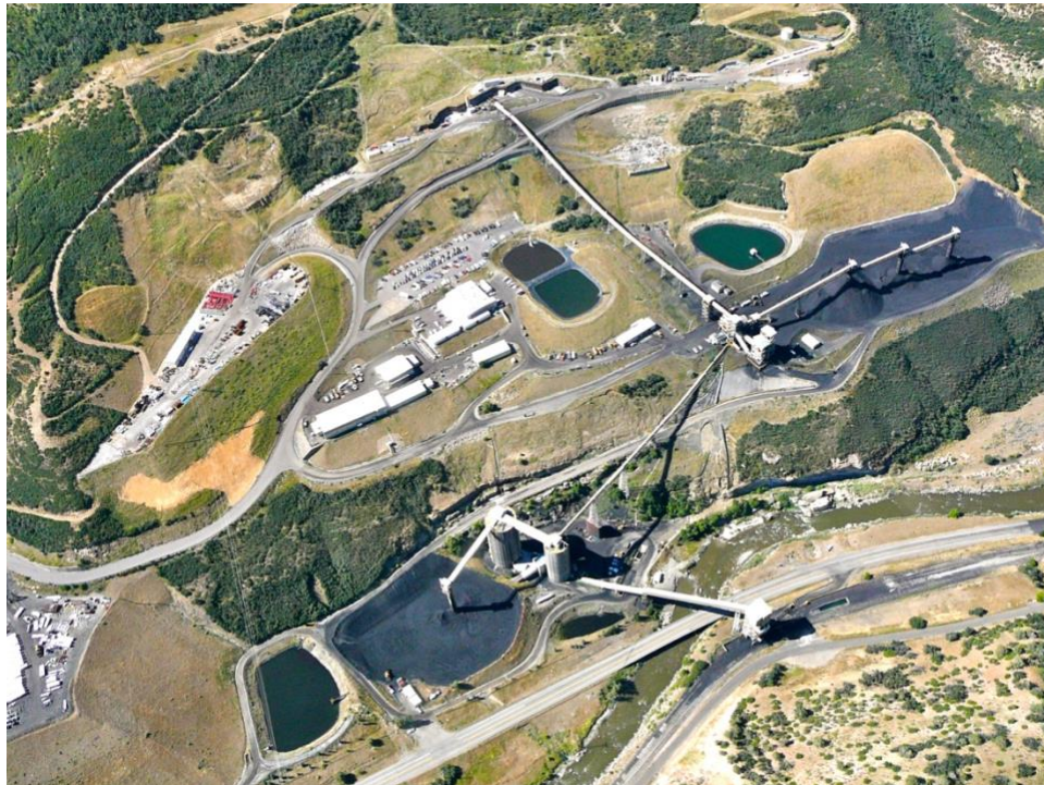
Figure 3: Aerial view of West Elk Coal Mine operations
