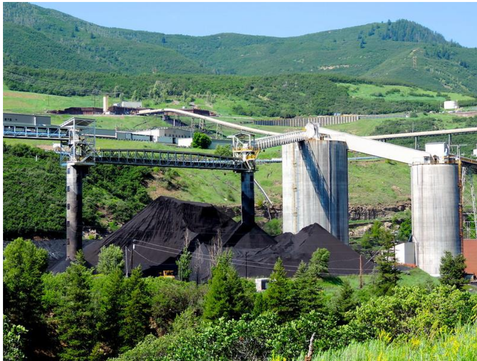
Figure 1: West Elk Coal Mine surface operations, including piles, conveyors, and silos
