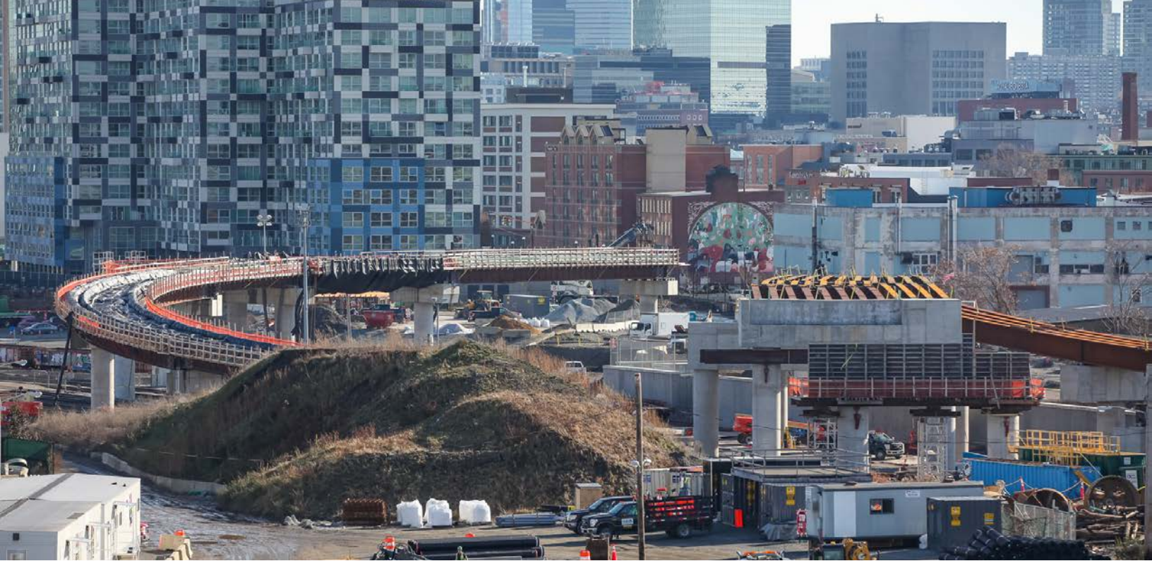
Figure 22: MBTA Green Line Extension. Photo by Weston & Sampson
