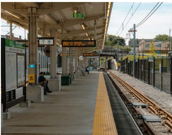
Figure 29: Platform for the Green Line Extension. Photo by Weston & Sampson
