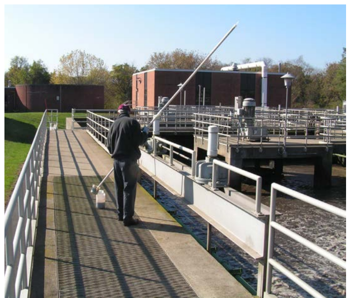
Wastewater Treatment Plant in Farmington Photo by Weston & Sampson.
