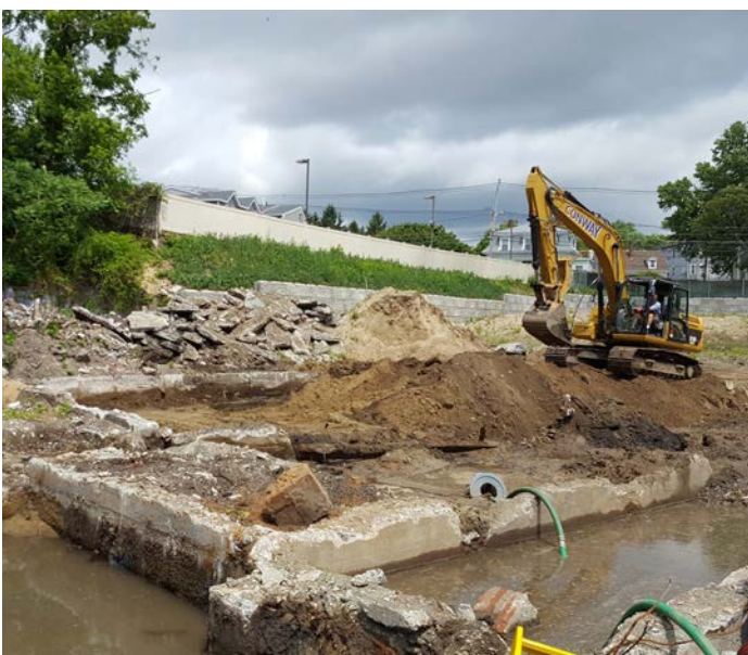
Tremont Crossing Brownfields Remediation. Photo by Weston & Sampson.
