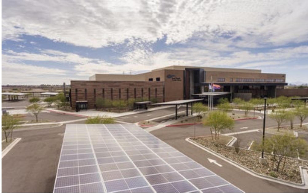
Figure 2. Solar parking canopies at SRPMIC’s River People Health Center (photo credit: Smith Group)
