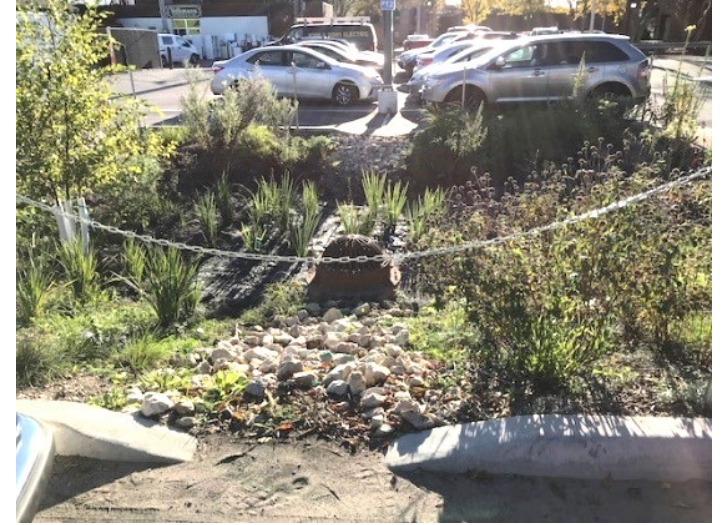
Parking lot infiltration MN Pollution Control Agency
