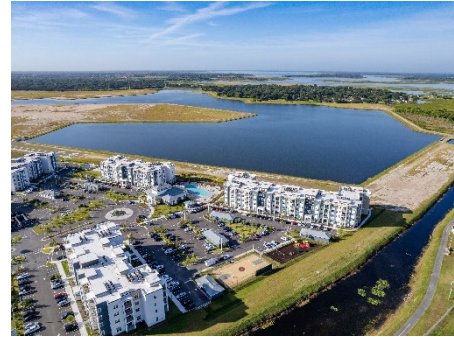
Photo credit: Toho Water Authority
