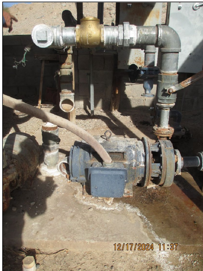
Photograph 12. There was one functional distribution pump, which showed signs of minor leaking. The other pump was fully removed at the time of the inspection.
