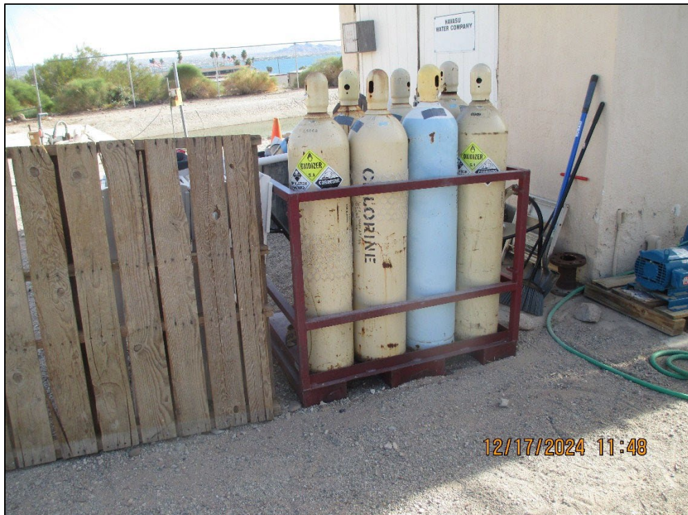
Photograph 14. Chlorine gas cylinders, even if most were empty, were stored in direct sunlight instead of indoors or under shade.
