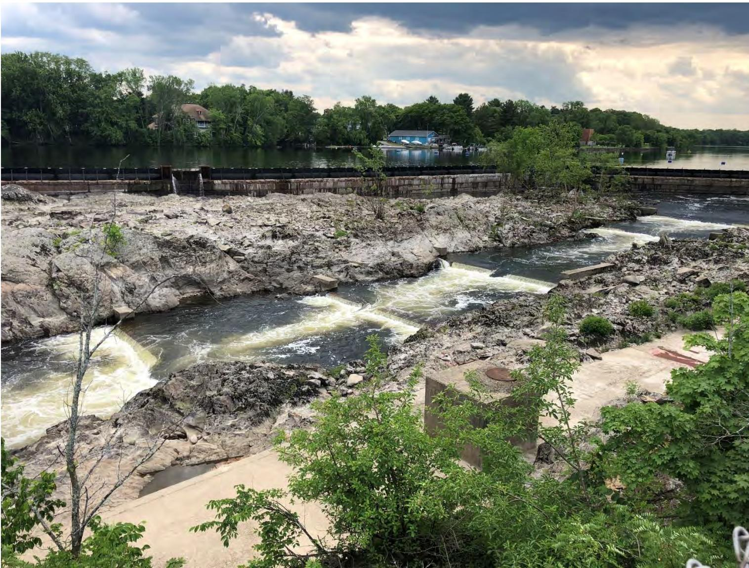
**Figure 2–3. Photo of the six concrete flow control weirs located within the Project bypassed reach and downstream of the entrance to the Pawtucket Dam vertical slot fishway.**
