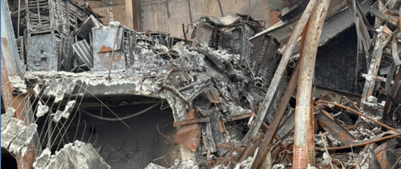
Due to the nature of batteries in different sections of the building, the battery removal process is split into two stages. With some initial stabilization and demolition, most intact batteries (above left) are accessible to recovery crews. The remaining batteries sit in the damaged portion of the building (above right), which will require additional demolition and debris removal work to access.
