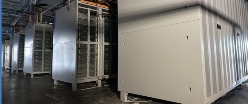
Due to the nature of batteries in different sections of the building, the battery removal process is split into two stages. With some initial stabilization and demolition, most intact batteries (above left) are accessible to recovery crews. The remaining batteries sit in the damaged portion of the building (above right), which will require additional demolition and debris removal work to access.
