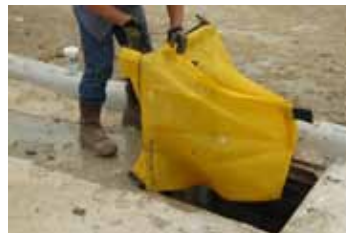
Slide Siltsack® over opposite side of grate.
