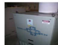
The MicoGen heat recovery system
