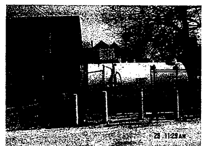
Figure 1-24 1,000-gallon gasoline AST between shop building and garage.
