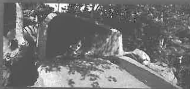
Storm Drain Outfall
