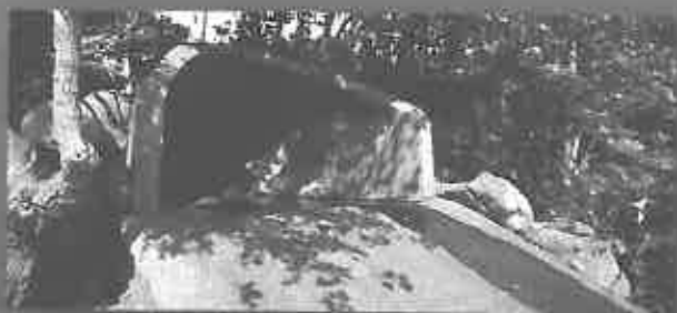
Storm Drain Outfall
