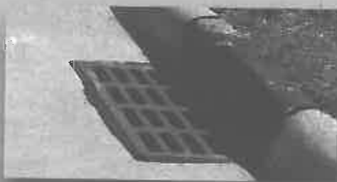
Storm Drain / Catcher outlet
