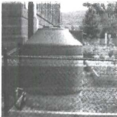
Cistern - Center Pepin Elementary School, Easthampton
