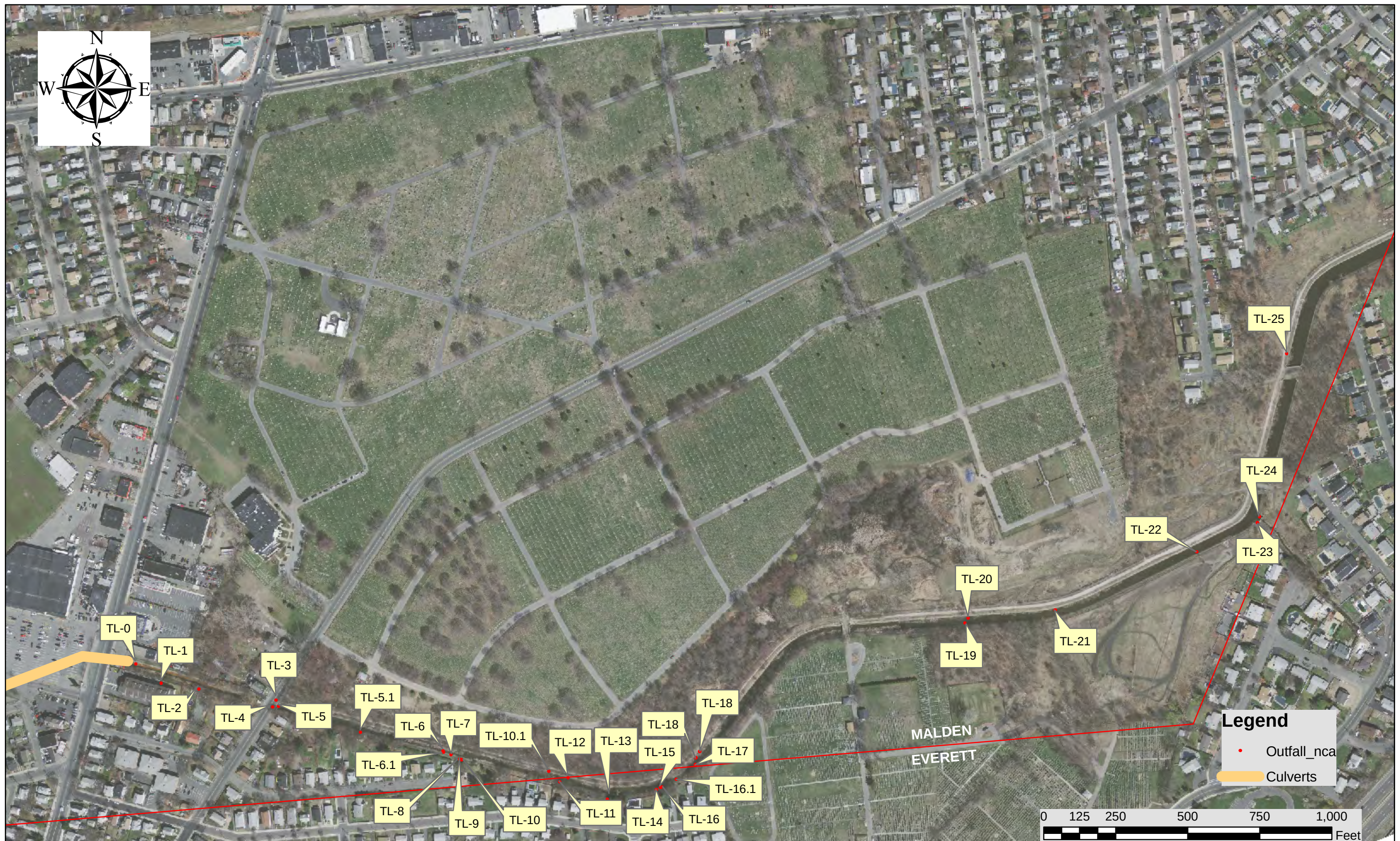
Figure 10 - Town Line Brook Outfalls
