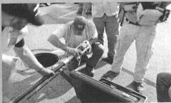
Sewer Operations technicians prepare a closed circuit TV camera to look for prohibited discharges such as fats, oils and grease.
