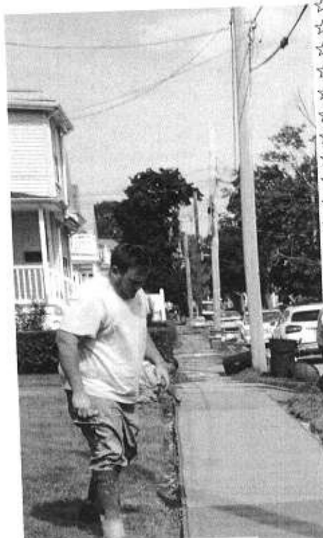
Side walk reconstruction in Wollaston.
