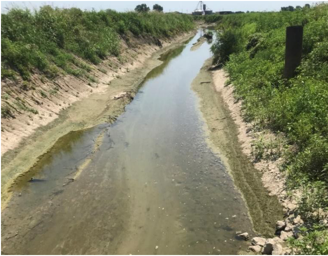
Figure 6: Ditch 32 Cash, AR before construction
