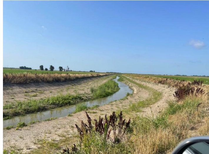
Figure 7: Ditch 32 Cash, AR after construction
