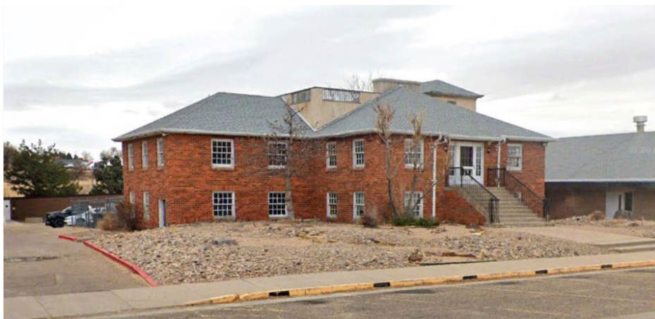
Figure 1. Sanitarium Building (Sans)
