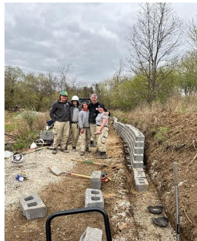
Figure 4. Trail Building Crew at Ohio River Islands NWR
